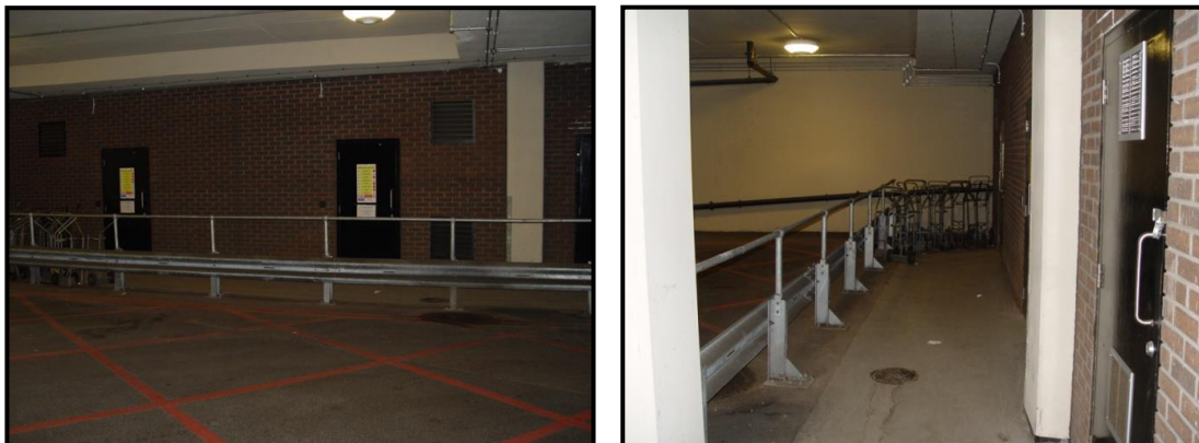
Figure 3 and 4: Example of traffic and vehicle management schemes to prevent unauthorised access to medical gas storage facilities.
