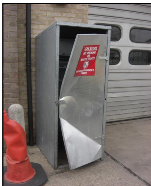
Figure 2: Example of poor storage which was exploited and cylinders stolen.
